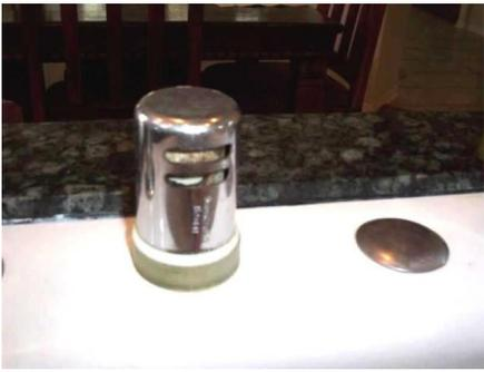
Figure 1. Dishwasher air gap at kitchen sink.
