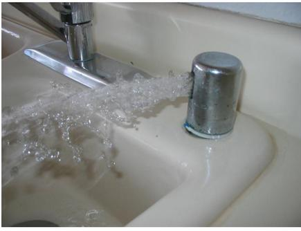
Figure 2. Dishwasher draining improperly through air gap.
